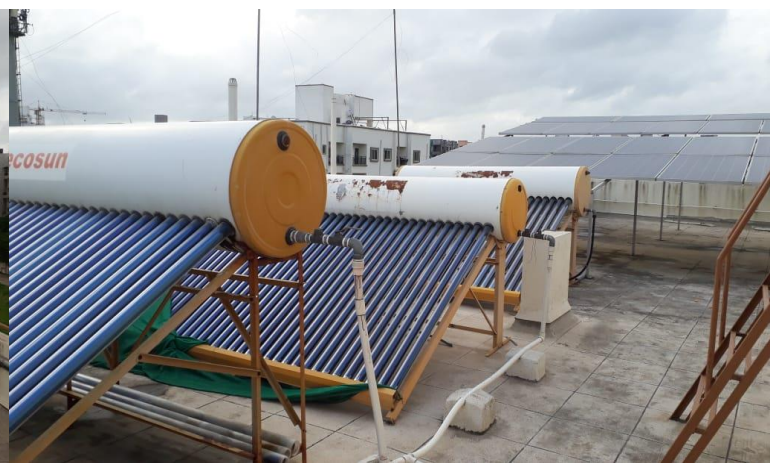
SOLAR PANELS for Electricity and water heating, Prerana Pune
